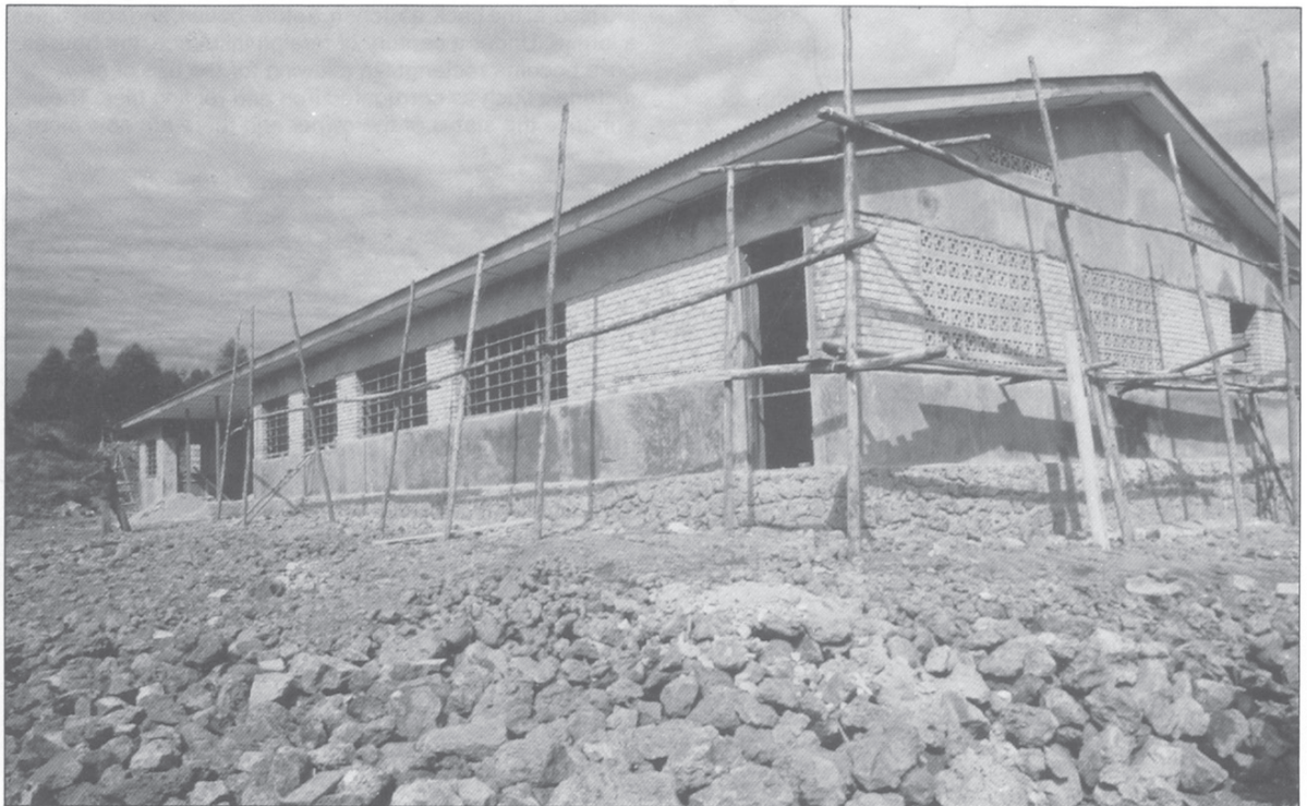
The new school building, using pozzolana-lime binder.
