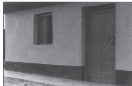
Improved finishing with pozzolana-lime rendering.
