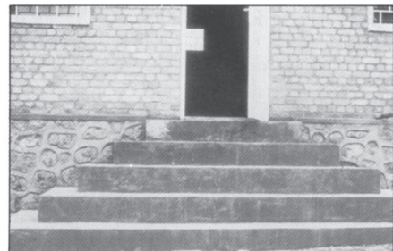
Application to stairs and base course.
