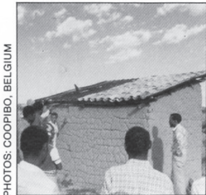
TARDEP demonstrates locally produced clay tiles on an improved mud-and-pole house.
