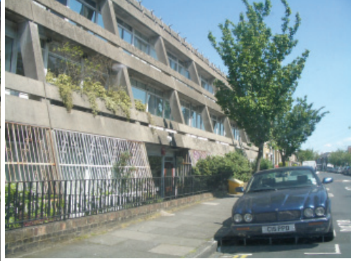
FIGURE 2.13 Existing building to be demolished on Calvert Road
