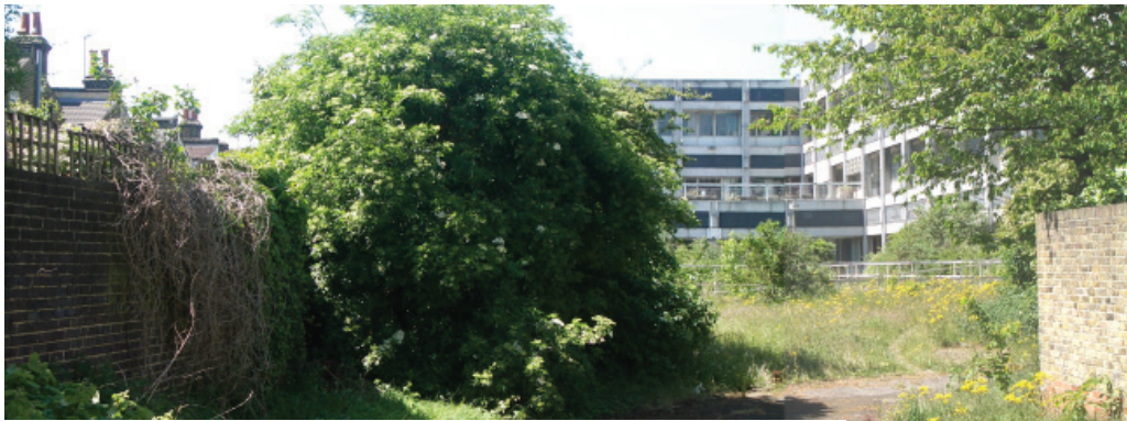
FIGURE 2.14 View of the former Hospital from Calvert Road entrance
