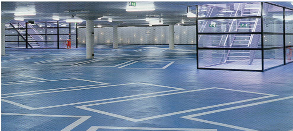
FIGURE 5.7.13 Underground parking with circulation cores to apartments above
