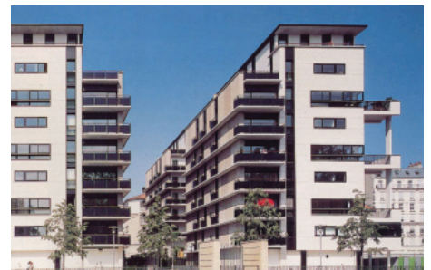
FIGURE 5.7.9 Gateway residential buildings
