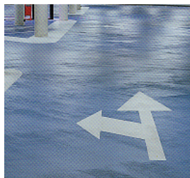
Underground car parking
