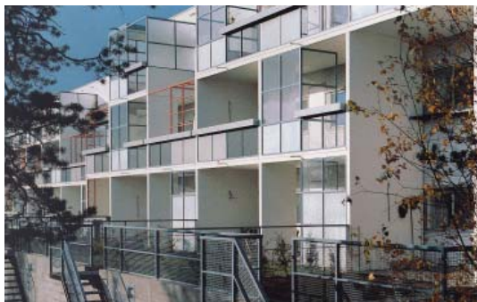
FIGURE 5.6.15 Outdoor terraces to apartments
