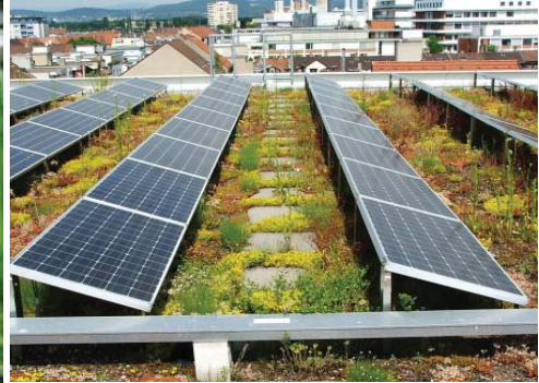
FIGURE 5.6.22 Green roofs with photovoltaics
